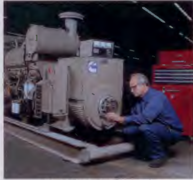
Motor Generator Overhauls
