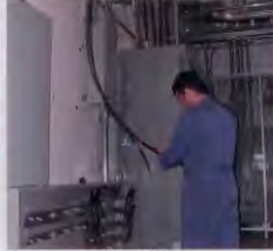
On Site Wiring
