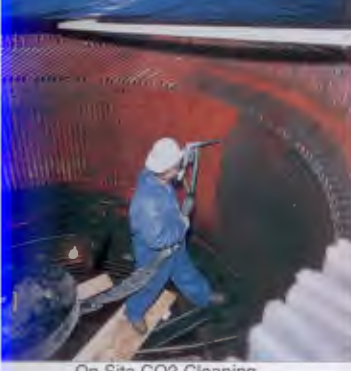
On Site CO2 Cleaning
